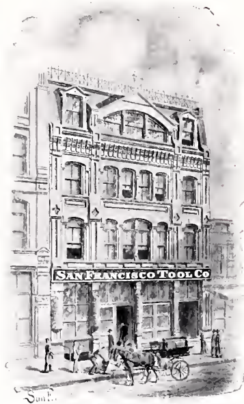
The Babcock & Wilcox Co., San Francisco Branch, San Francisco Tool Company.
